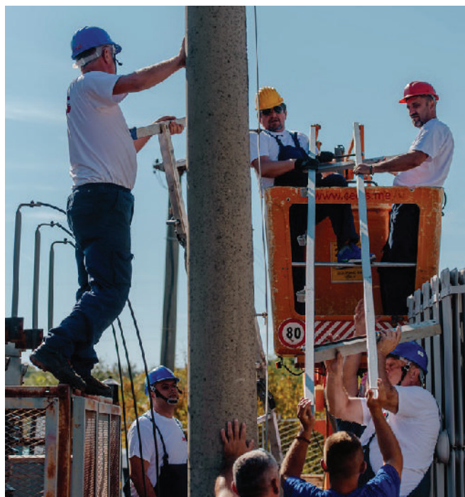
Remont TS "Barutana"
