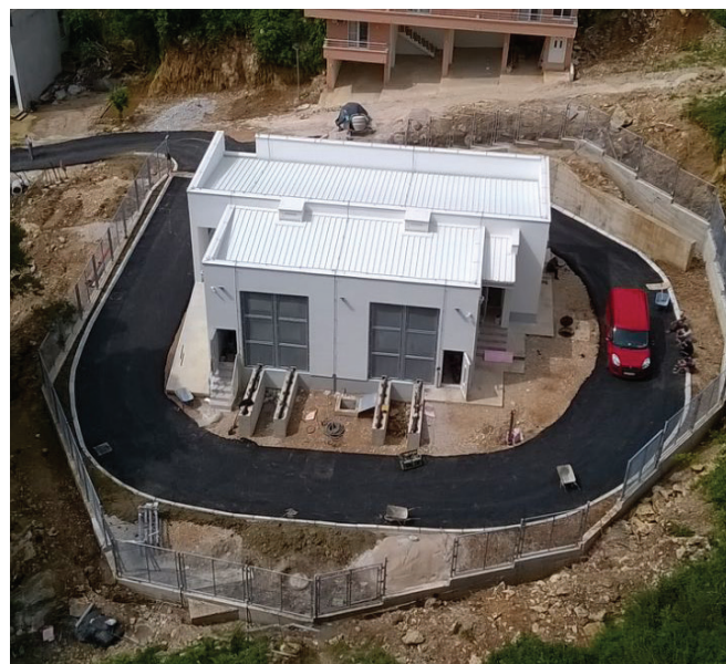
TS 35/10kV "Novi Ulcinj"
