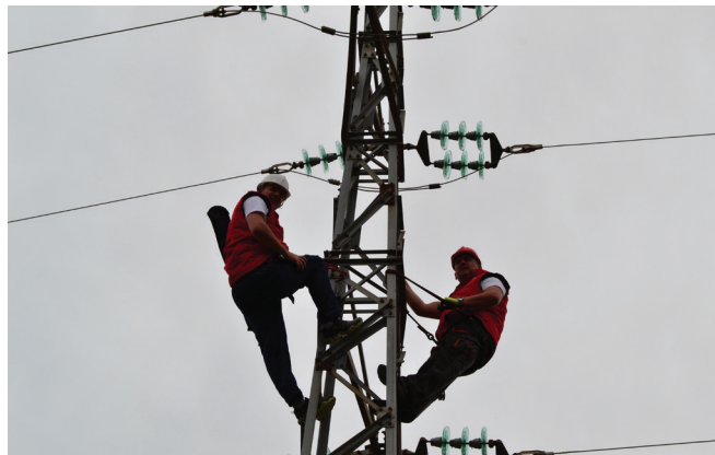
Remont 35kV dalekovoda u Ostrosu
